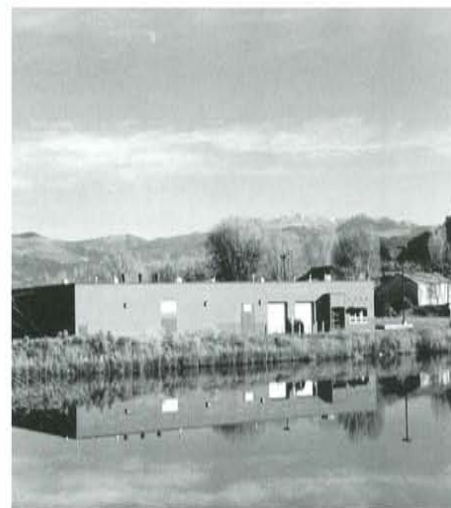
The CWRPDA assisted the Town of Eagle in funding this wastewater treatment plant through the Clean Water 1997 Series A bond issue.
