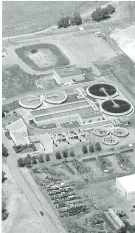
Funding for the Sand Creek Wastewater Reuse Facility was obtained through the Water Pollution Control Revolving Fund.
